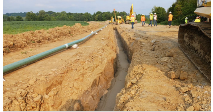
Gas Pipeline Construction
