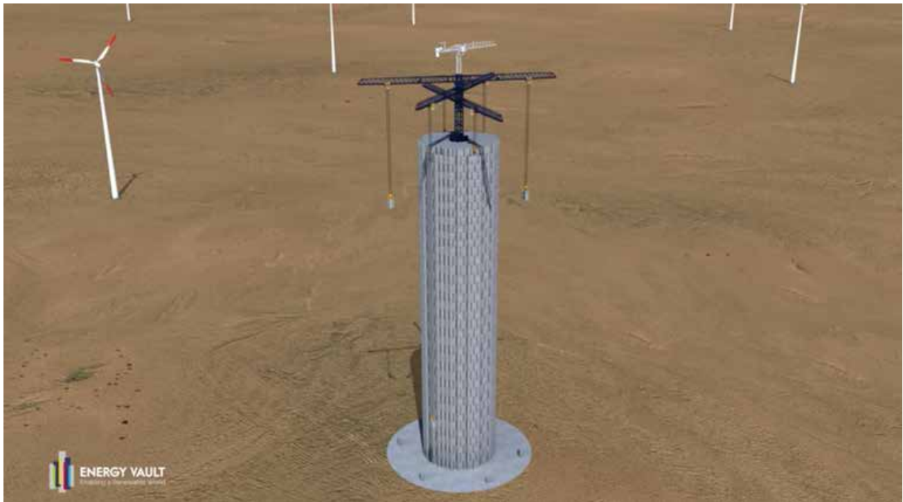
Figure 6.12-7: Concrete Block Energy Storage Diagram 71
